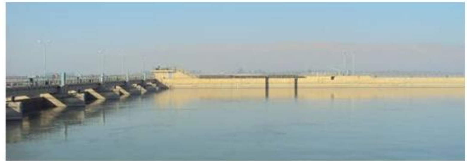
View Upstream of the Chashma Barrage
