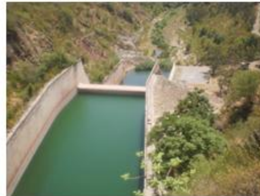
Spillway Stilling Basins
