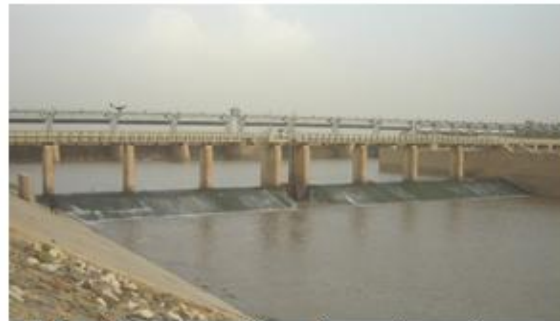
Islam Barrage - View from downstream side
