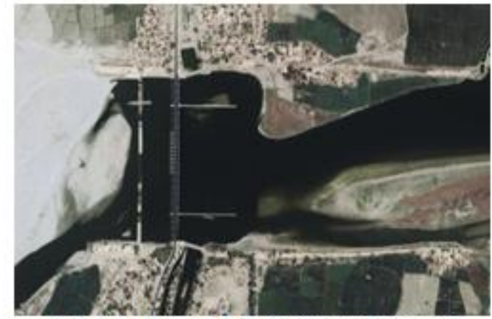
Aerial View of Existing Barrage
