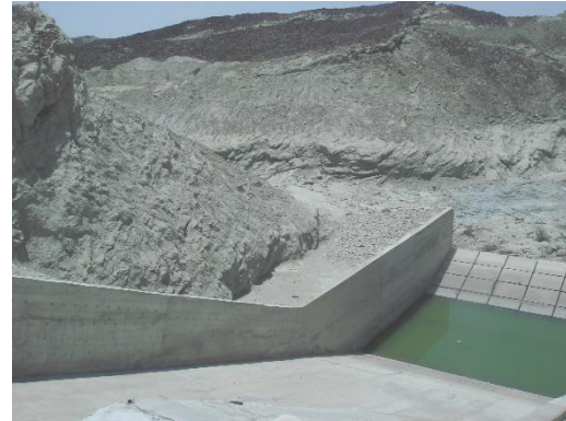
Main Spillway Flip Bucket
