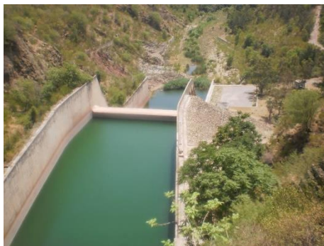
Spillway Stilling Basins
