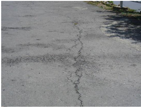
Crack on Dam Crest
